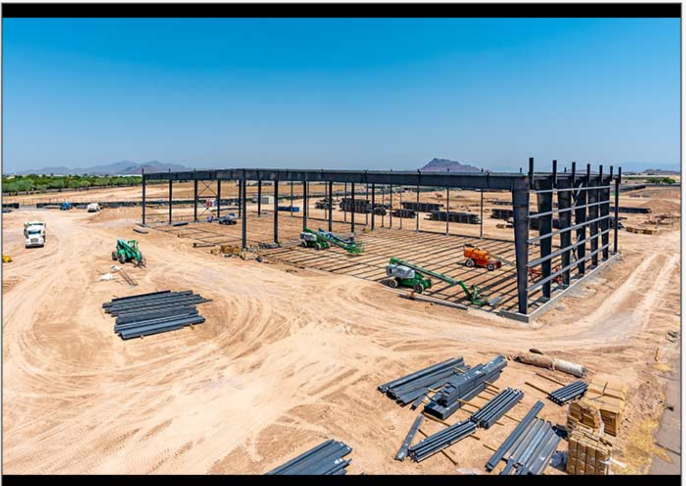
MESA HANGAR AT FALCON FIELD AIRPORT
