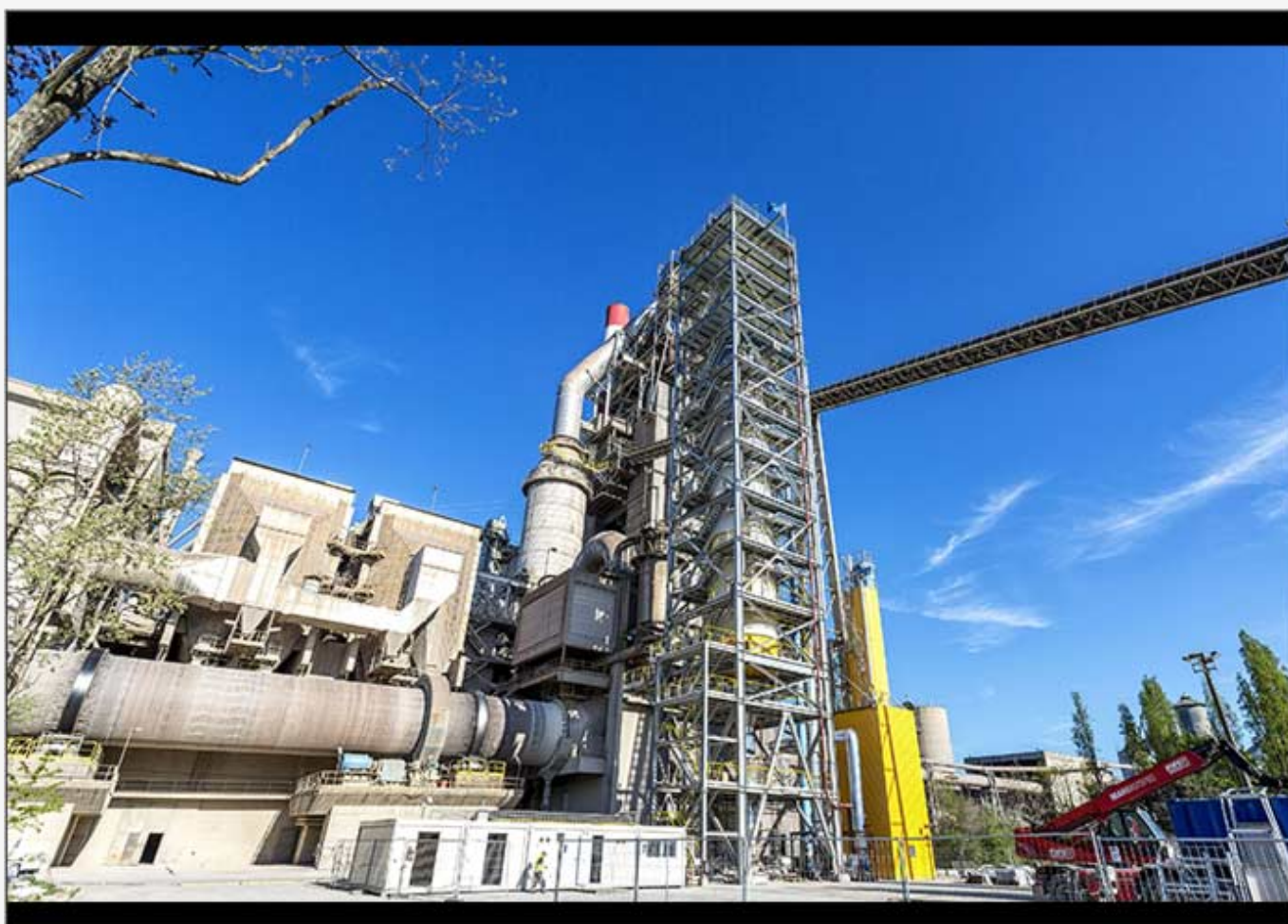
CALIX DECARBONISING TECHNOLOGY AT THE LEILAC PLANT
